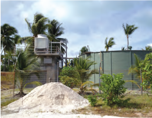
Water pumping and storage infrastructure at the Bonriki groundwater reserve, South Tarawa.
